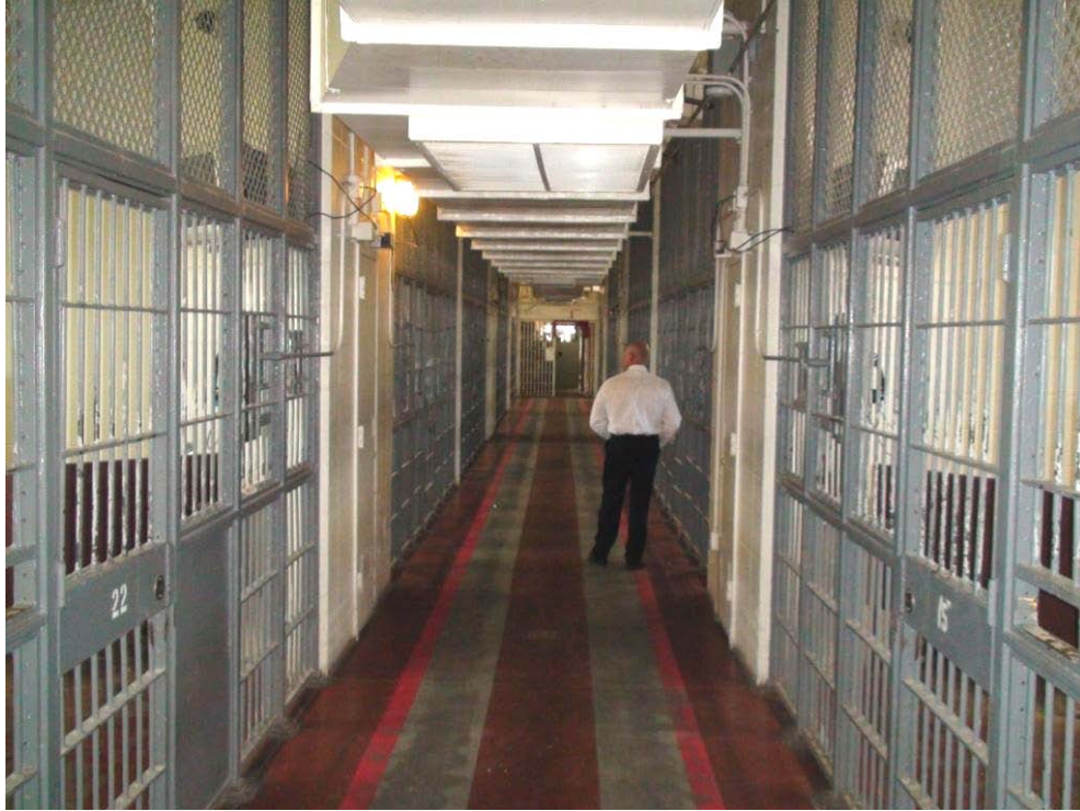
Roger Bauman Facility (RBF) Linear Housing Unit Circulation Corridor
