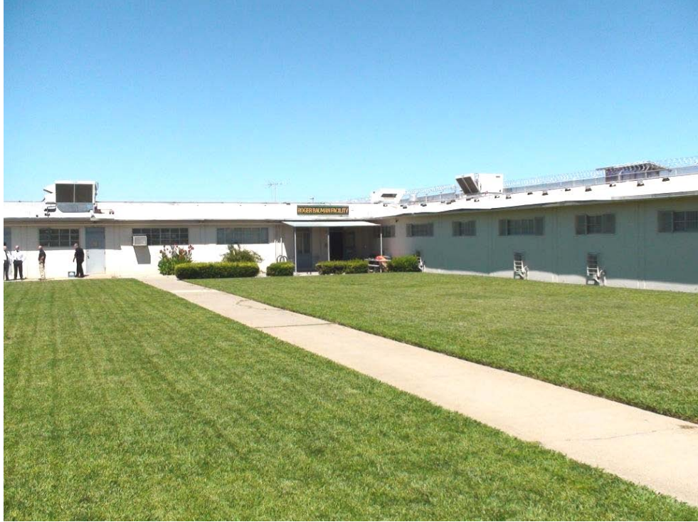
Roger Bauman Facility (RBF) Housing Unit Entry
